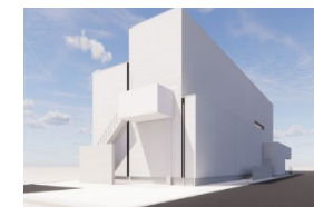
S-RAMCO Line 2 (under construction)
