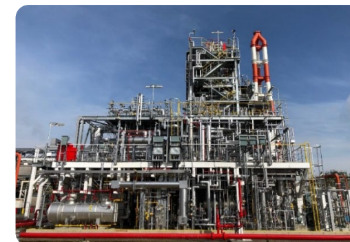
Test equipment for manufacturing ethylene derived from ethanol
